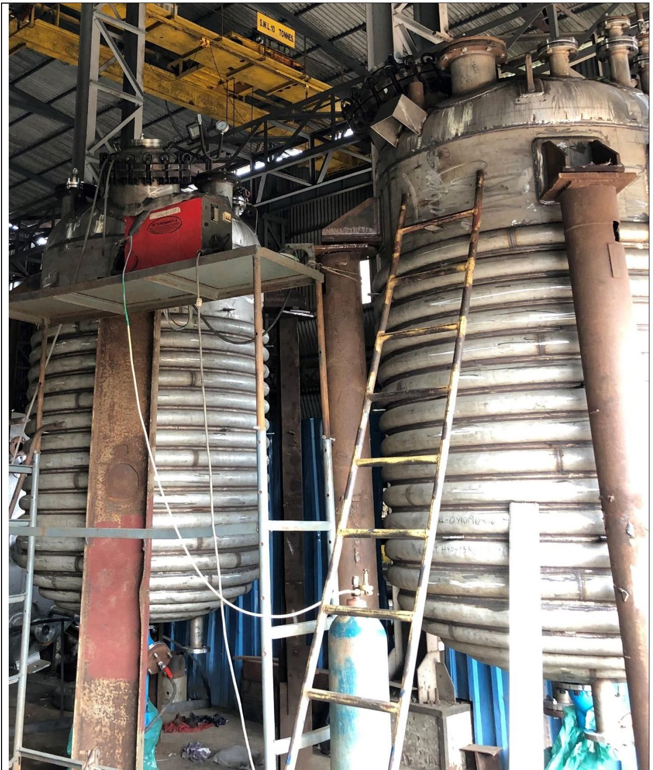
REACTOR TESTING IN WORKSHOP
